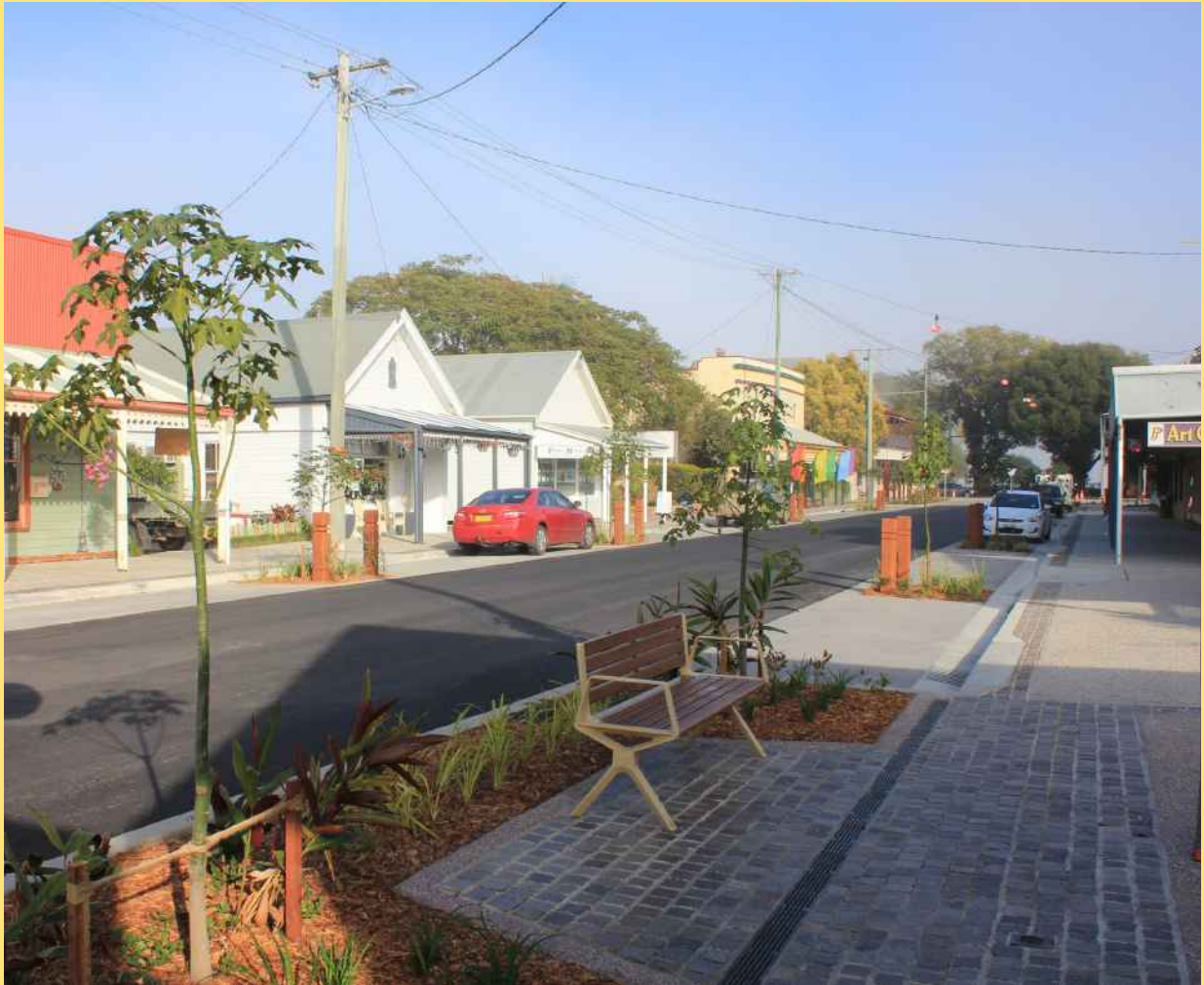
Ulmarra High Street Upgrade Project, NSW
