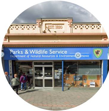
Clear glazing, Main Street REALMstudios
